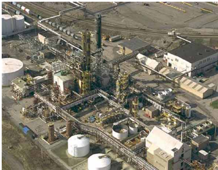
An aerial view of the ring chlorination isomer columns that we purchased and assumed responsibility to remove from the site. (Niagara Falls, NY)
