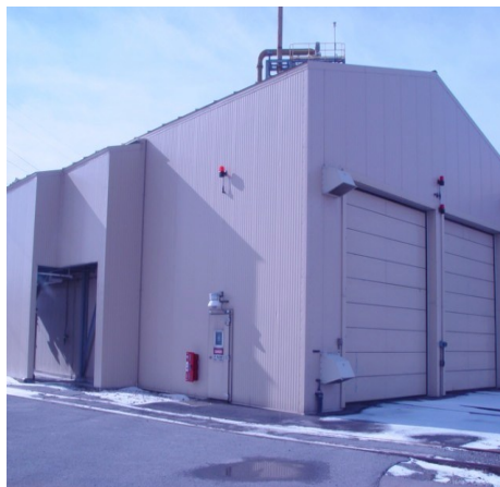
90 ton HF tank car two bay unloading plant with a devoted building, built 1998. This is one of the nine closed processes that enabled us to perform the project at no cost .
