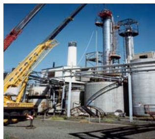
Our crew dismantles a 140 ft. distillation column
