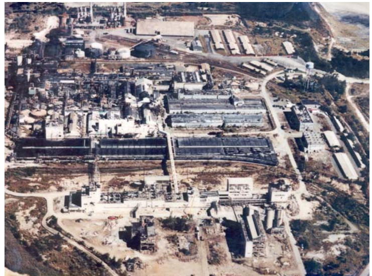
Aerial view of the complete 150 acre NL Industries Sayreville, NJ site that we decommissioned.
